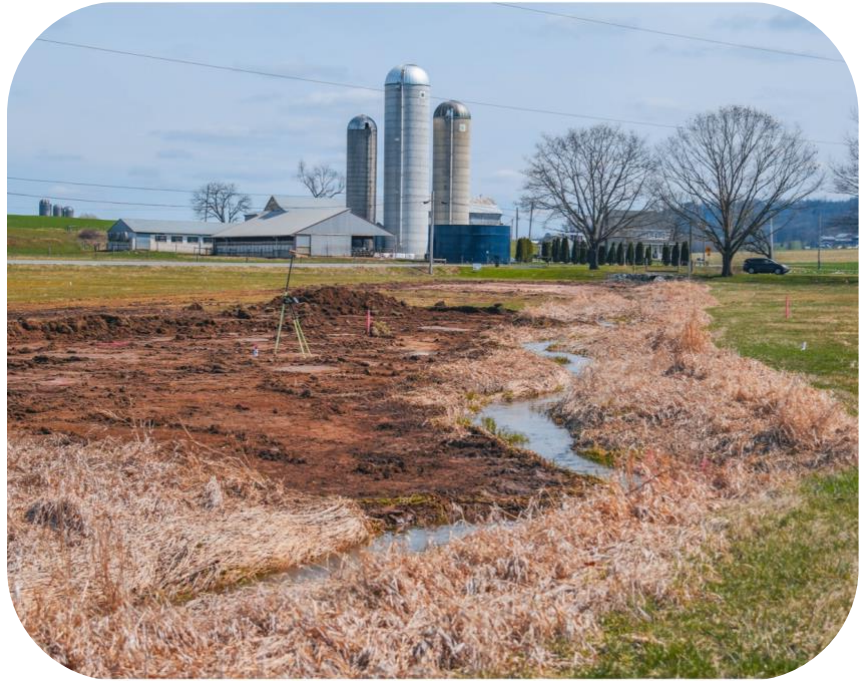
Floodplain Restoration Construction in PA ©The Nature Conservancy
