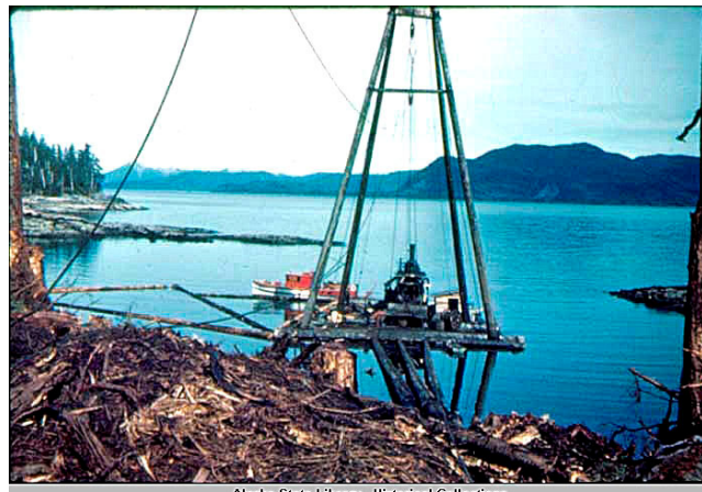
FIG 2. A-frame logging with a steam donkey along the shoreline of Edna Bay on Kosciusko Island northwest of Prince of Wales Is. Circa 1940s. Most of the shoreline with productive forests in Southeast has received some level of timber harvest. (Alaska State Library, Dora Sweeney, P421-301)
