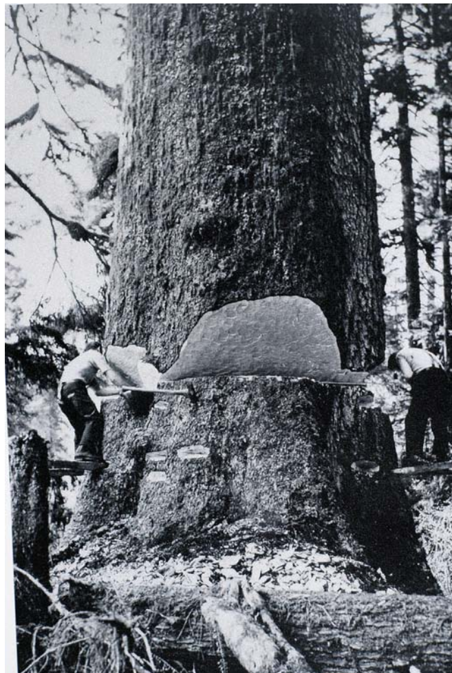
FIG 1. Hand loggers using spring boards to stand on and axes and hand saws to cut a large old-growth Sitka spruce in the southern Tongass circa 1900. The biggest, best quality, and most accessible trees were cut first throughout the forest. (USFS historical photo)
