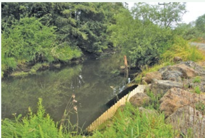
Figure 6. A road and culvert crossing a tributary of Coos Bay.
