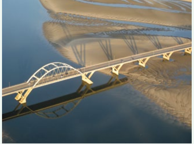
Figure 16. The Alsea Bay bridge places little impact on the estuary's connectivity.
