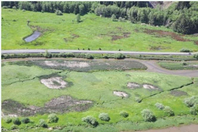
Figure 4. A road on fill intersecting the Umpqua estuary.
