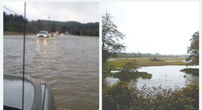
Figure 9. Restoration at Circle Creek Ranch. The left-hand photo shows flooding on Hwy. 101—south of Seaside, Oregon—prior to the removal of berms along the Necanicum River. The photo on the right shows flooding in September 2013 after berms had been removed, allowing the floodwaters to access the floodplain at natural bank elevations. The floodplain was completely inundated but the highway was not.
