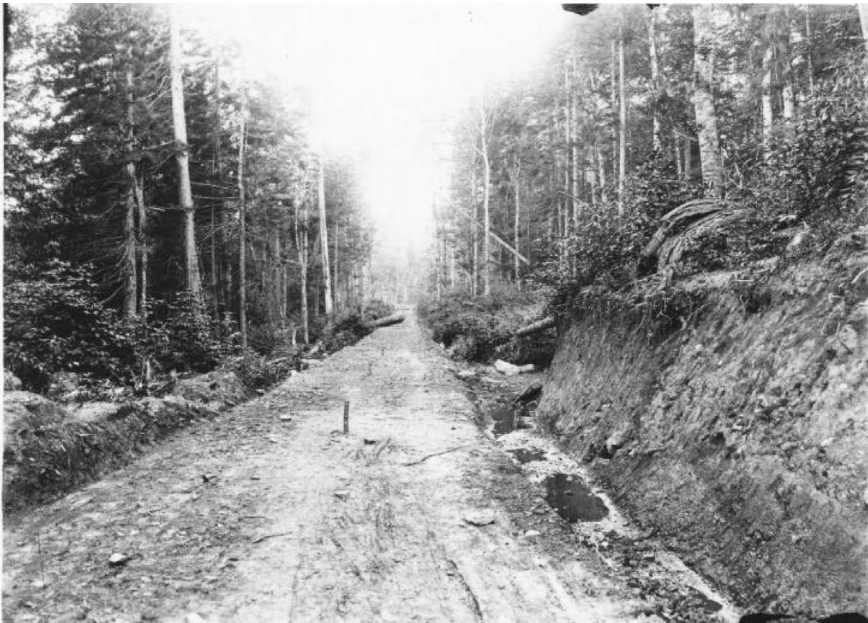
Fig. 5.1 Construction of a railroad grade near Cranberry Glades, Pocahontas County, West Virginia, around 1911. Photo by USDA Forest Service
