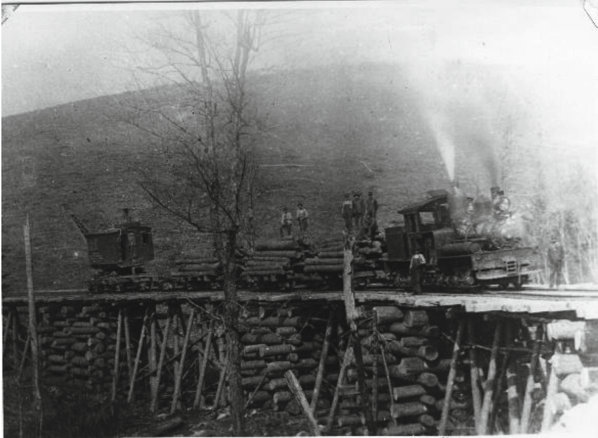
Fig. 9.1 A steam loader on a Shay engine, 1910 (photo by USDA Forest Service)
