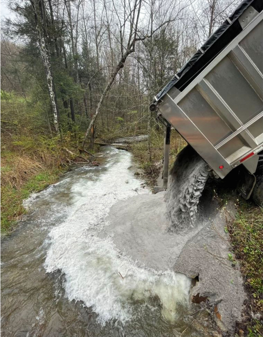
Fig. 6.3 Application of crushed limestone into a headwater stream impacted by acid deposition. Photo by Eric Gladwell
