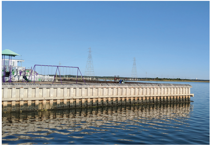
This vinyl bulkhead in Wildwood, NJ, is an example of a conventional gray shoreline stabilization project. © The Nature Conservancy
