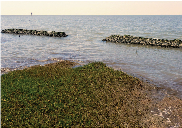
Three years after construction, vegetation re-established behind the oyster reef breakwater at Gandys Beach. © The Nature Conservancy
