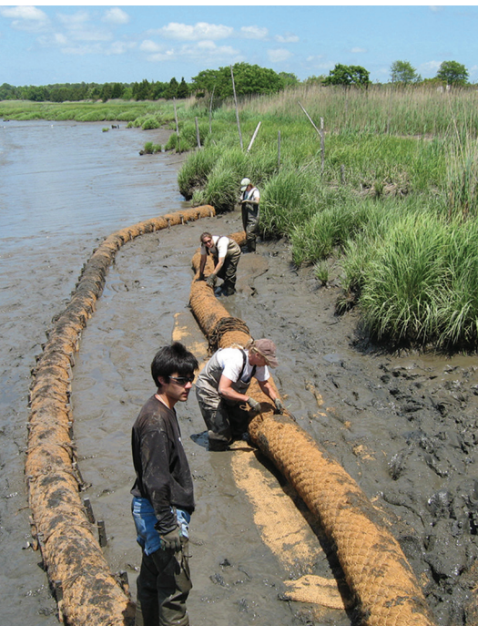
Construction of Matts Landing coir roll living shoreline. © Partnership for the Delaware Estuary
