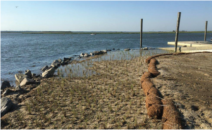
Strathmere: Coir roll terraced slope and water-ward rock sill
