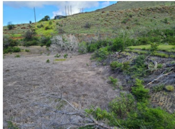
Figure 48: Ukumehame Reservoir 2. Photo: DLNR, Dam Safety Program
