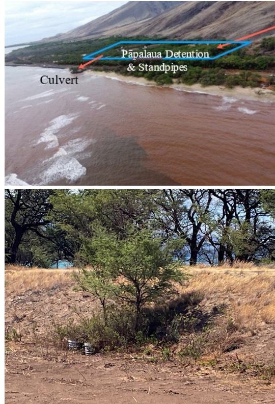
Figure 44: Pāpalaua Detention Basin and culvert locations. Photo: DOFAW
