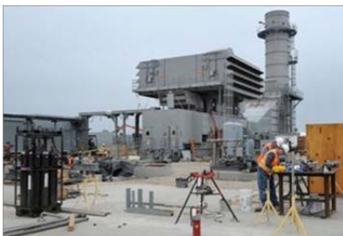
Edison Peaker Plant under construction
