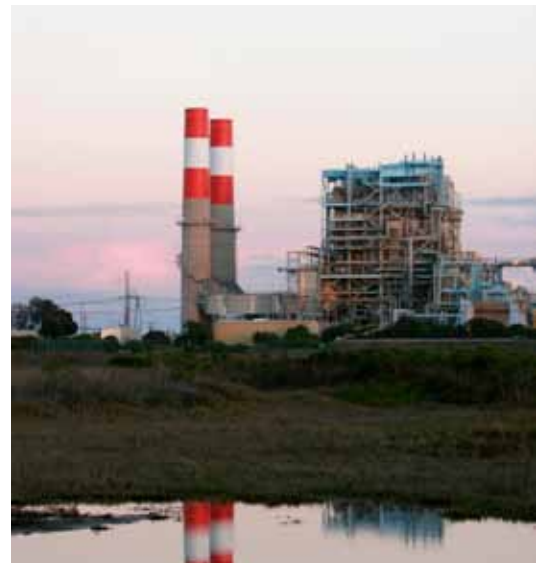
Vulnerable coastal infrastructure in Oxnard, CA
