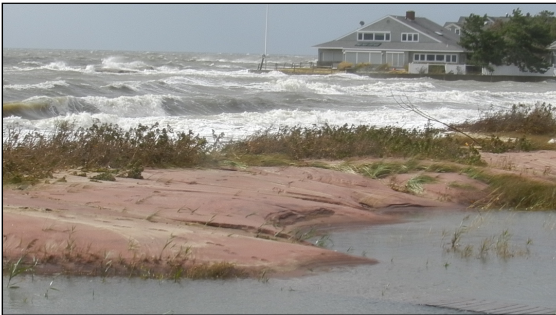
Natural Infrastructure defending the coast against waves during Storm Sandy (Madison, Connecticut) © Adam Whelchel/TNC
