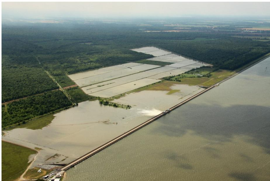
**Figure 8.** The Morganza Spillway (long line in center) during the 2011 Mississippi Flood. The Morganza Spillway was opened during this flood, allowing the Mississippi River, on right, to begin to flow into the Morganza Floodway (fields and forests on the left).
