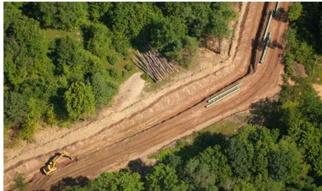
Activities associated with all forms of infrastructure development, including shale gas, such as ground clearing and construction for roads and pipelines (as pictured above), present risks of erosion and sedimentation. © *The Nature Conservancy* (Mark Godfrey)
