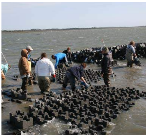
Volunteers constructing oyster reef from Oyster Castles near Box Tree. Photo by Bowdoin Lusk
