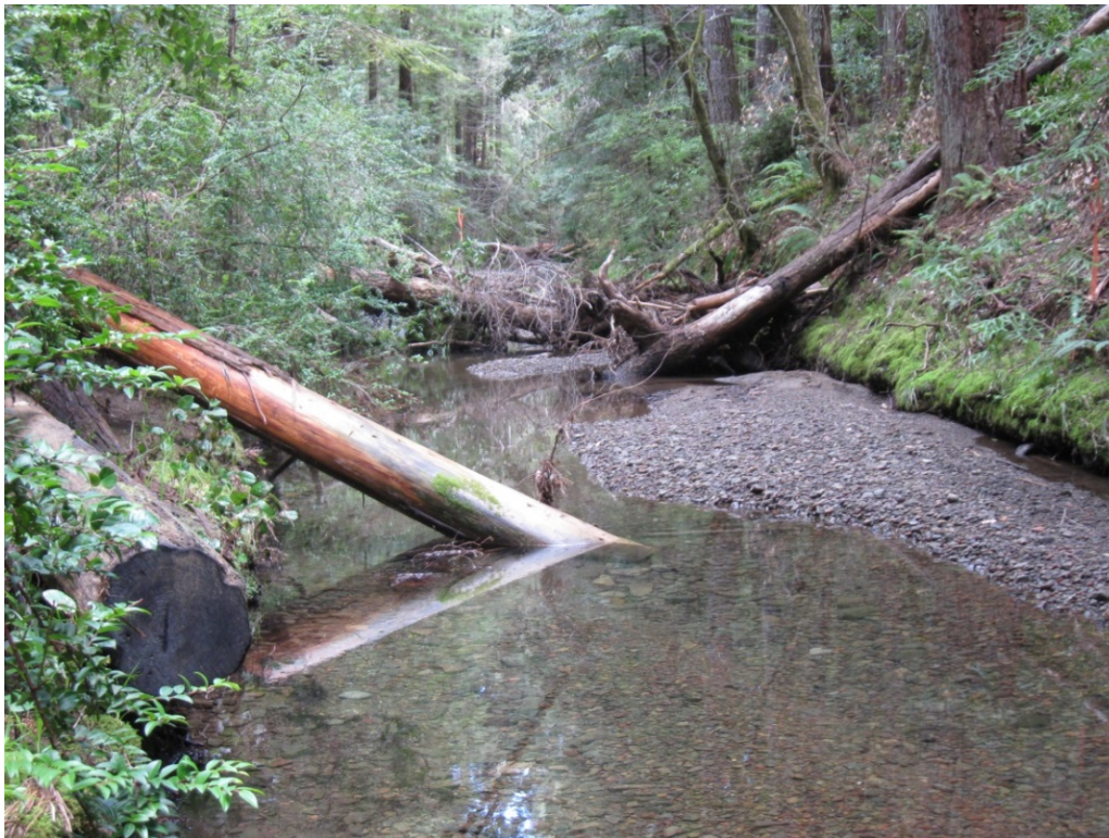
Figure 9. View of anchored wood structures installed in 2012 by CCC crews in the North Fork of the South Fork Noyo River on Jackson Demonstration State Forest.
