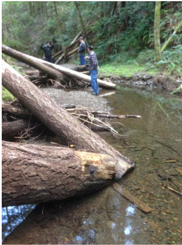
Figure 10. Anchored structure at NFSF Noyo River (photo: Jonathan Warmerdam, NCRCRWQB)
