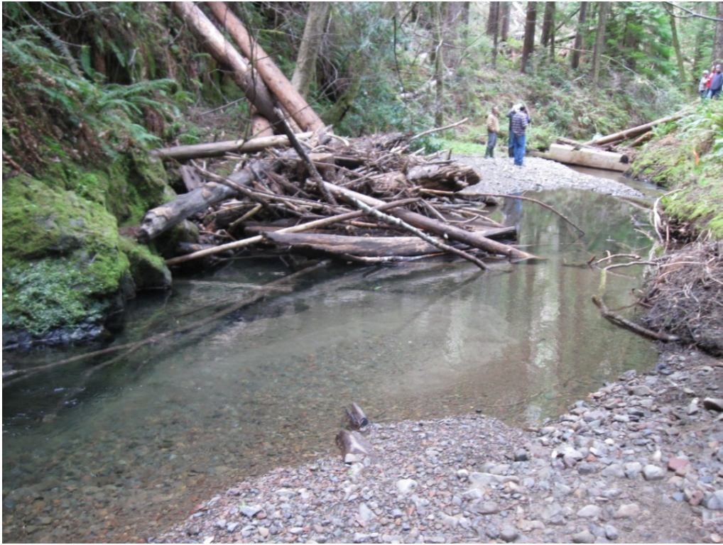
Figure 6. North Fork of the South Fork Noyo River—instream large wood project with traditional anchoring, implemented in 2012 by CCC crews from Ukiah. Considerable wood has collected on the original structure.
