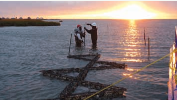
Workers prepare a site for installing ReefBLKtm, a proven technique for growing oyster reefs. ©Amy Smith Kyle.
