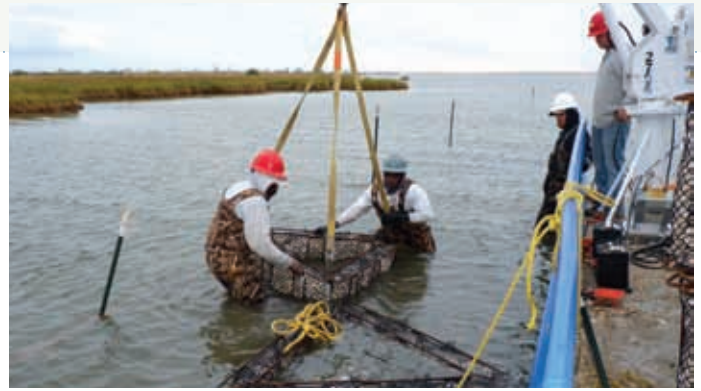
ReefBLKtm, interlocking steel cages filled with recycled shells, are being used in Louisiana and other Gulf states to grow oyster reefs. ©Amy Smith Kyle
