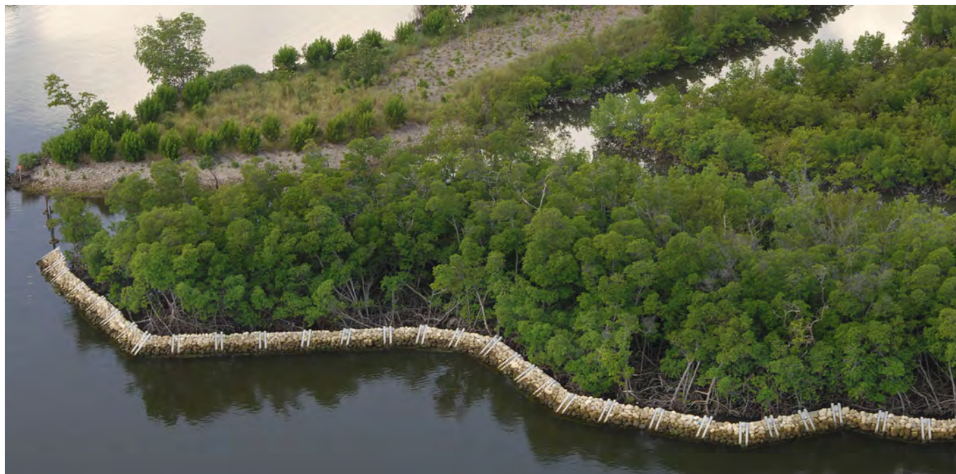
Riprap crib mangrove hammock close up ©Paul Krashefski, Broward County, EPCRD, 2011
