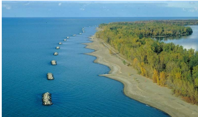
Figure 9: Typical Breakwater Project
