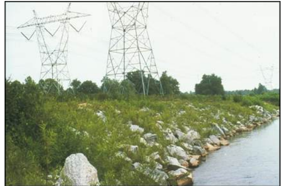
Figure 8: Typical Joint Planted Revetment
