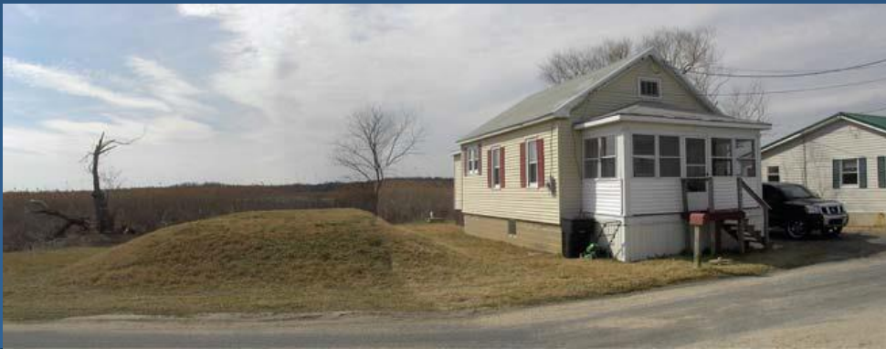
Elevated septic system from “Rolling Easements,” EPA
