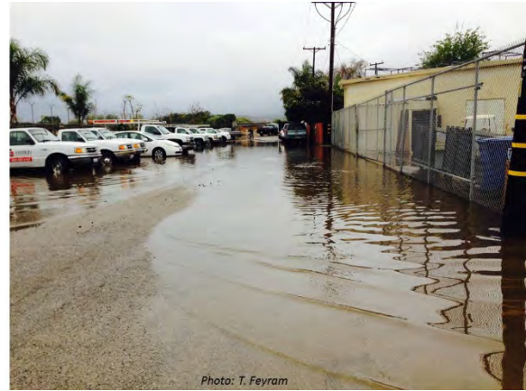
Photo 3-3. Flooding in the Placencia Neighborhood 2014 (Photo: T. Feyram)
