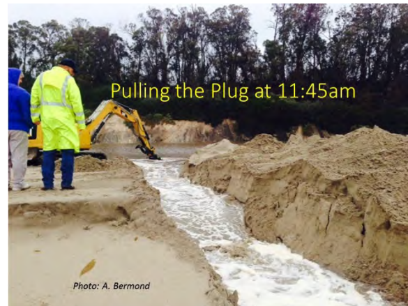
Photo 2-3. Goleta Slough Inlet Breaching, 2014 (Photo: Patrick Bermond, City of Santa Barbara)
