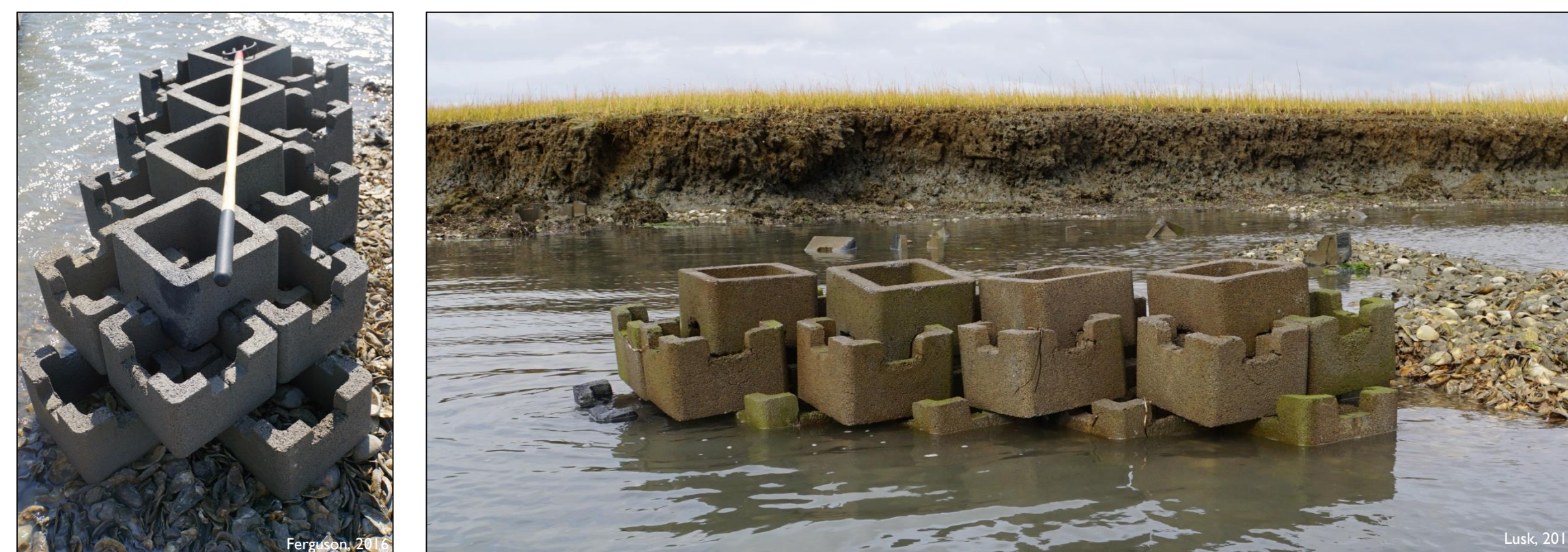
Figure 1. Typical constructed oyster reef design used in Virginia's coastal bays composed of interlocking bio-concrete blocks.
