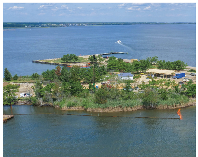
A living shoreline was constructed at Berkeley Island County Park. © T&M Associates
