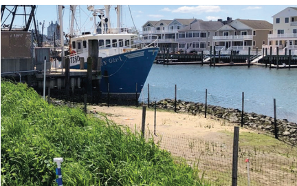
Gardner's Basin: Rock sill with planted grasses
