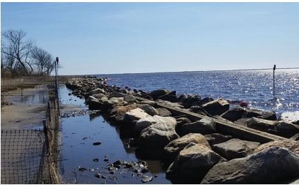
Berkeley Island: Rock sill with wooden bulkhead spine
