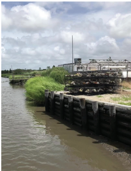
Side by side living shoreline and wooden bulkhead at Mats Landing. © Stevens Institute of Technology
