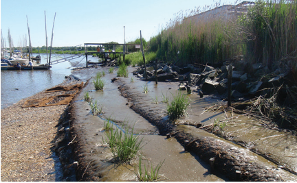
Matts Landing: Coir roll marsh edge protection
