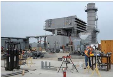
Edison Peaker Plant under construction
