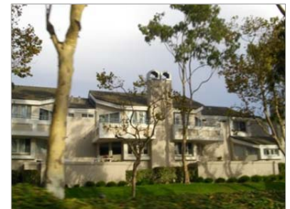
Some projects in Port Hueneme are built atop fill
