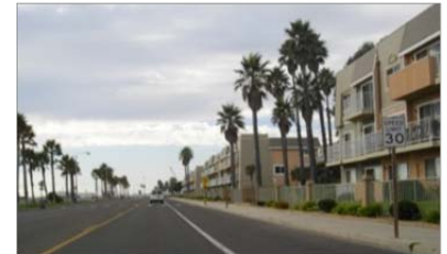
Surfside Drive was designed with consideration for rising sea levels
