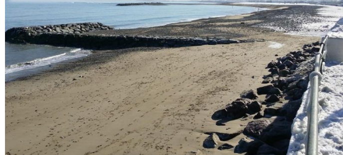
Winthrop Shores, Winthrop, MA Photo courtesy of Applied Coastal Research & Engineering
