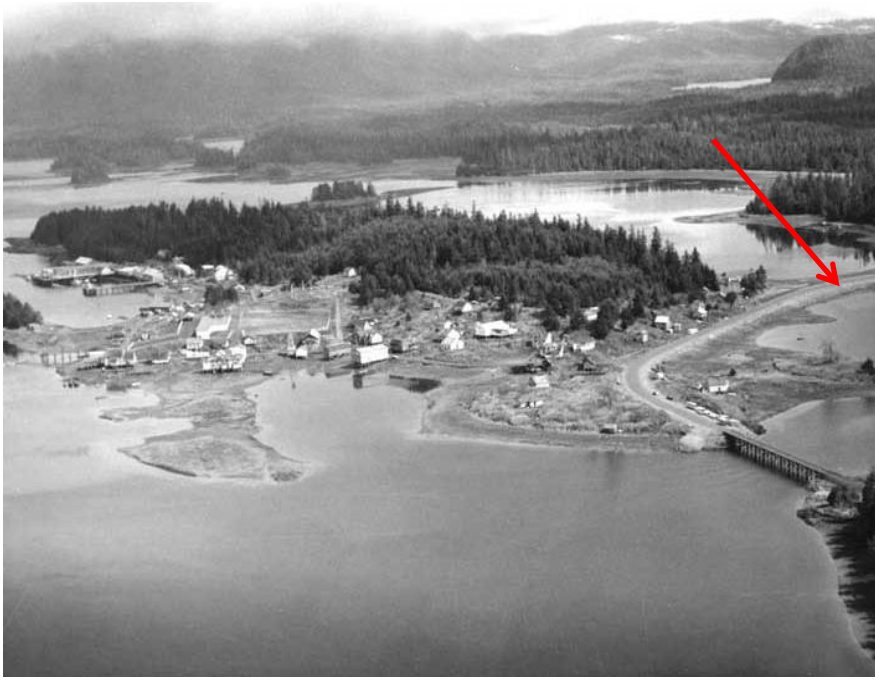
Figure 2: (After) This aerial photograph shows construction of a road in 1964 through the corner of the village, and over a bridge, one of the two exits from the estuary. The previous exit is above and on the right side of the photo, where you can see the road goes along what became a causeway: an elevated road (marked by the red arrow). Photo: Aaron T. Isaacs, 1964
