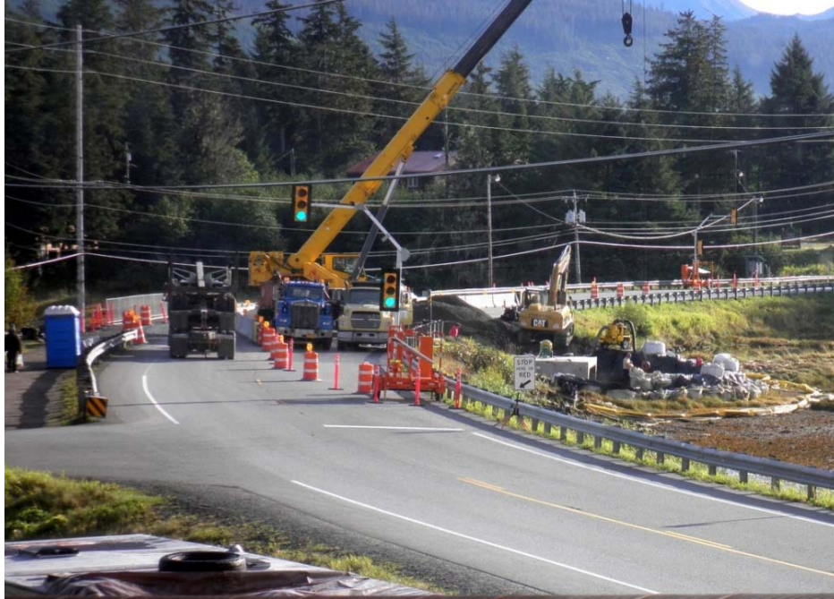
Figure 7: Construction underway on culvert beneath highway. Photo Credit: The Nature Conservancy, 2011
