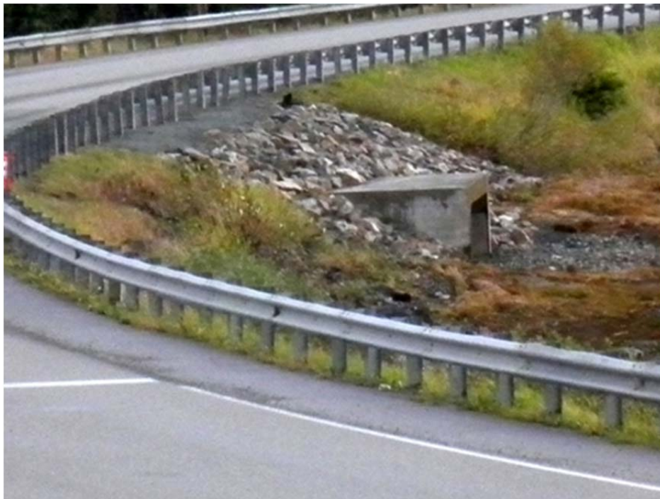
Figure 8: Photo of completed culvert at low-tide. Photo: The Nature Conservancy, 2011
