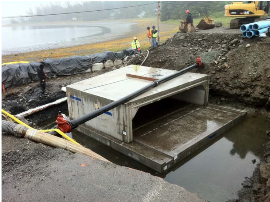
Figure 14: The culvert and utility lines. Photo: The Nature Conservancy, 2011.
