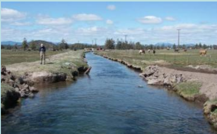
Large irrigation diversions
