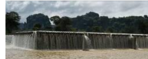
Aeration Weir to improve quality of the released water – comprehensive water monitoring
