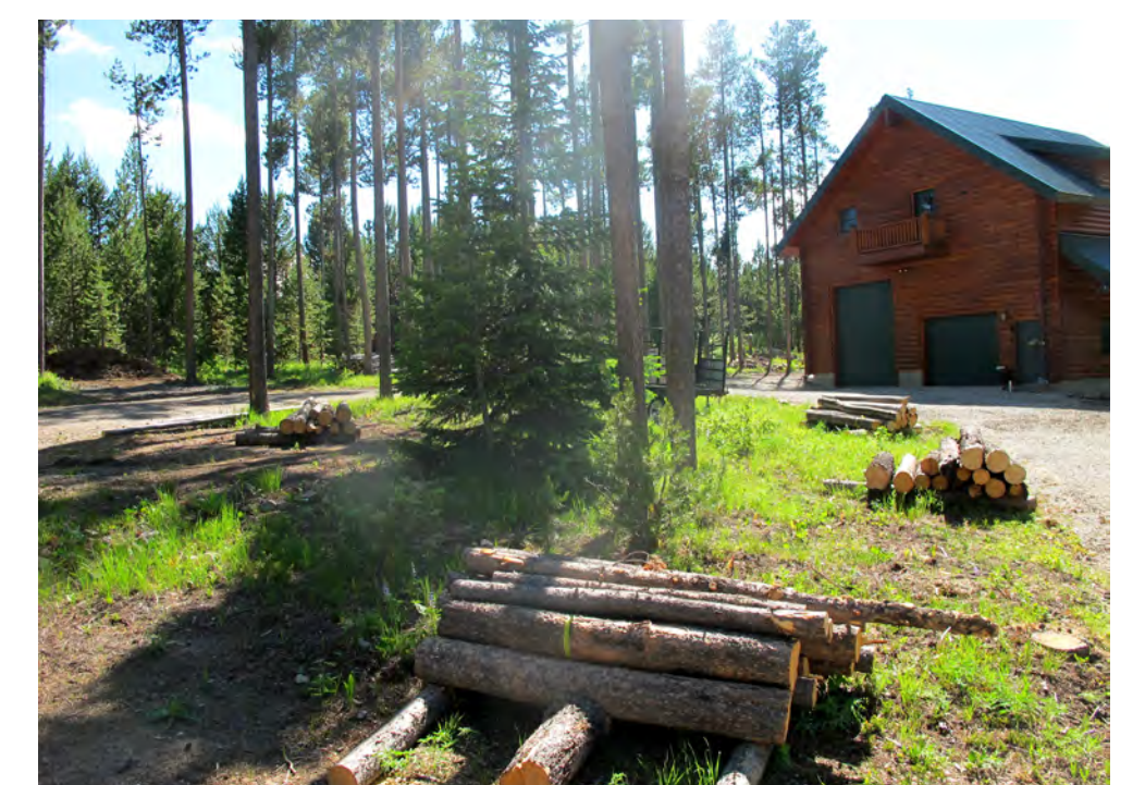
Fuels were cut and ready for removal at one of the four defensible space demonstration projects completed by the Island Park collaborative in 2014. Photo: Jessica Simpson
