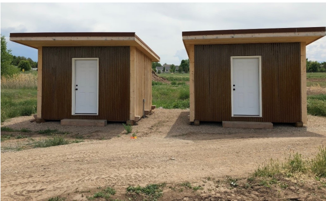
Two sheds involved in an experiment at USU Botanical Center, Kaysville. Shed built with CLT is on the left. Photo by Jerry Goodspeed.
