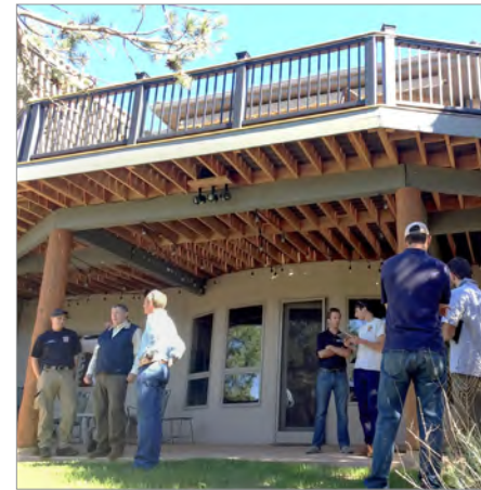
Participants in the Fire Adapted Colorado (FACO) learning exchange discuss potential issues with decks, as part of the larger conversations about assessing hazards and planning mitigation efforts.
