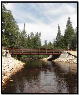
In 2011, the Conservancy replaced three culverts where the CCI Road crosses the South Branch of the Two Hearted River. Previously, excess water would flow over the road, washing debris and sediment into the river. The new 45-foot bridge is reducing sedimentation by 9.8 tons per year and connecting up to 24 miles of stream.
