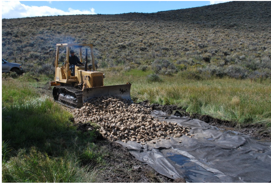
Building low water crossing on Wolf Creek Ranch
