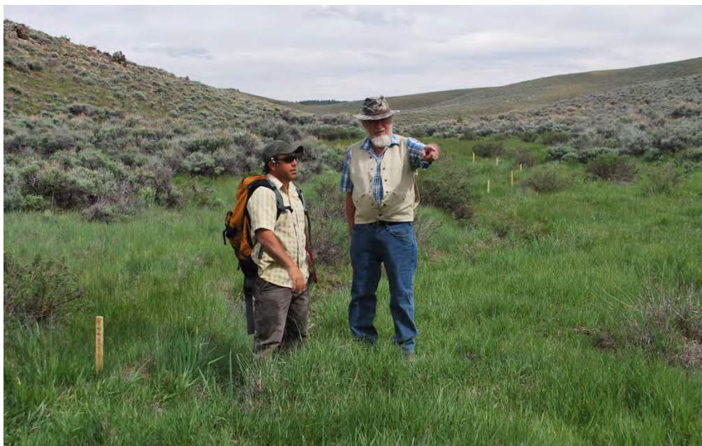
26. Team members and restoration experts Shawn Conner, BIO-Logic, Inc. (left) and Bill Zeedyk, Zeedyk Ecological Consulting discussing placement of rock structures in Chance Gulch.
