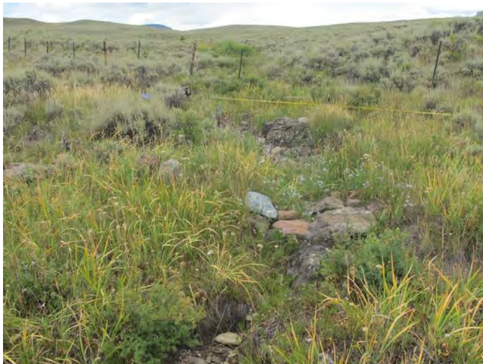
32, 33. Picture taken shortly after installation and one year later showing positive response to a Zuni bowl (above near fence), built to control a head cut, and a one rock dam (below), built to capture sediment to raise the bed of the channel, and recruit vegetation on West Flat Top Mountain on US Forest Service lands.
