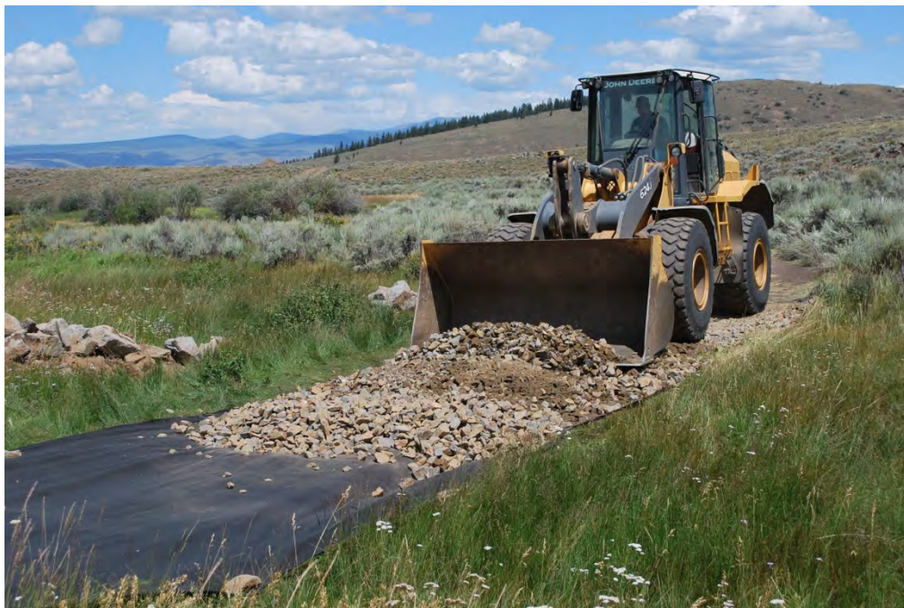
8. Gunnison Gravel front-end loader builds a low water crossing at Chance Gulch, August 2014.
