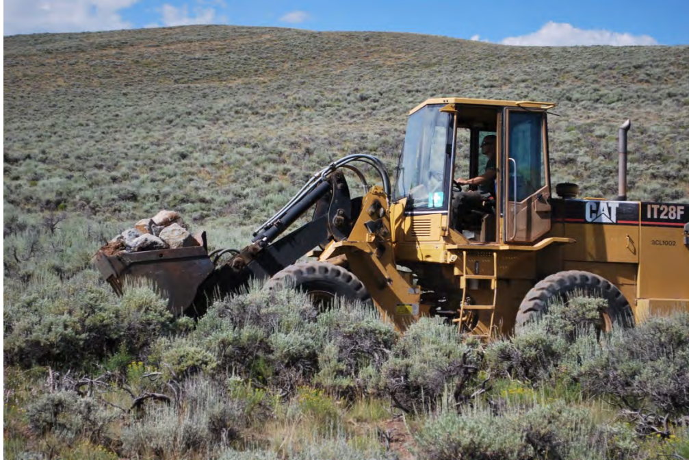
7. Gunnison Gravel delivering rock to staging area at Chance Gulch, July 2014.
