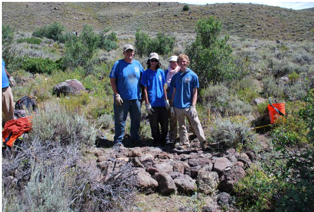
14. Western Colorado Conservation Corps field crew complete one rock dam structure at West Flat Top Mountain on US Forest Service lands above Redden Ranch, consisting of locally collected volcanic rock, August 2014.
