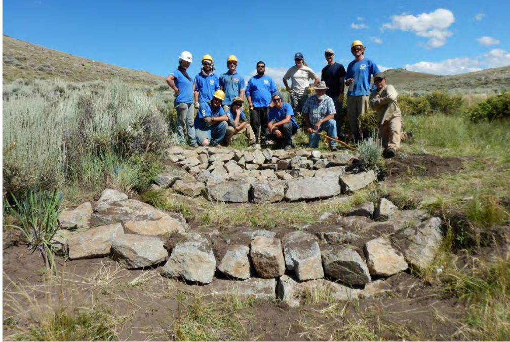
13. Western Colorado Conservation Corps, Nathan Seward, Colorado Parks and Wildlife, Bill Zeedyk and Shawn Conner, BIO-Logic celebrate completion of a Zuni bowl (below crew) with one rock dam (foreground) at Chance Gulch, August 2014.
