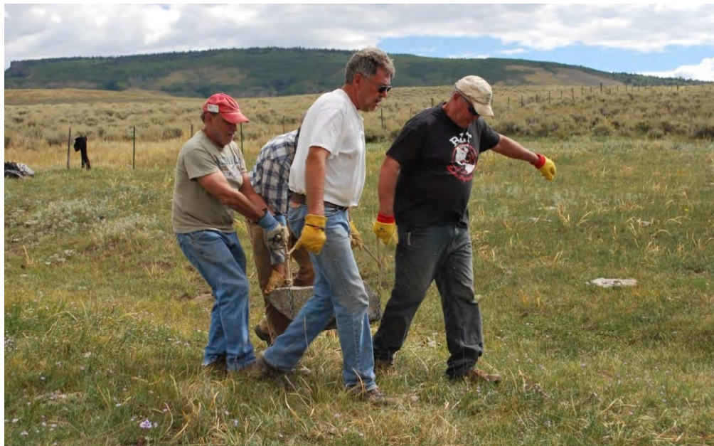
18. Wildlands Restoration Volunteers Crew Leader Mark Flower hauls rock with help of volunteers on West Flat Top Mountain, US Forest Service lands, September 2014.
