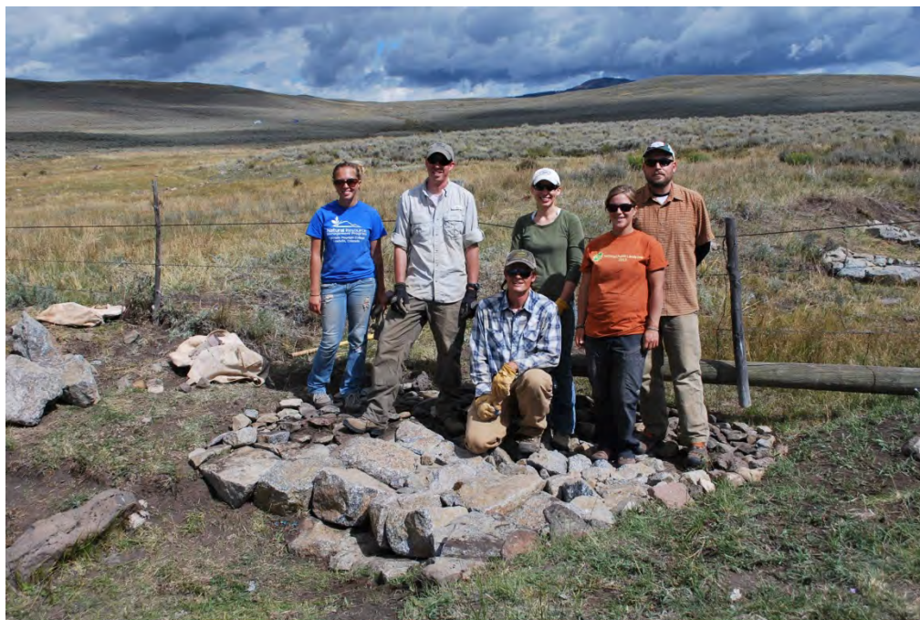
20. Wildlands Restoration Volunteer Crew Leader Clayton BonDurant (low center) and volunteers complete Zuni bowl to control a head cut on West Flat Top Mountain on US Forest Service lands, September 2014.
