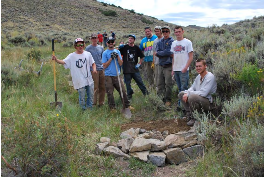
21. Western State Colorado University Ecological Monitoring class completes a one-rock dam in Chance Gulch, directed by Nathan Seward, CPW (in background).
