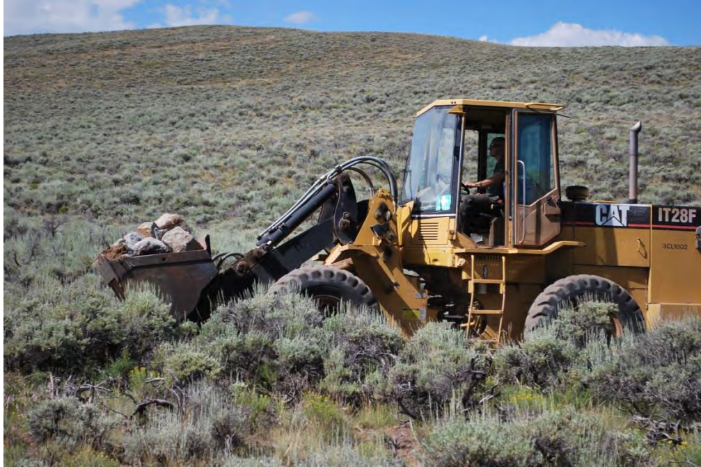
9. Gunnison Gravel delivering rock to staging area at Chance Gulch, July 2014.
