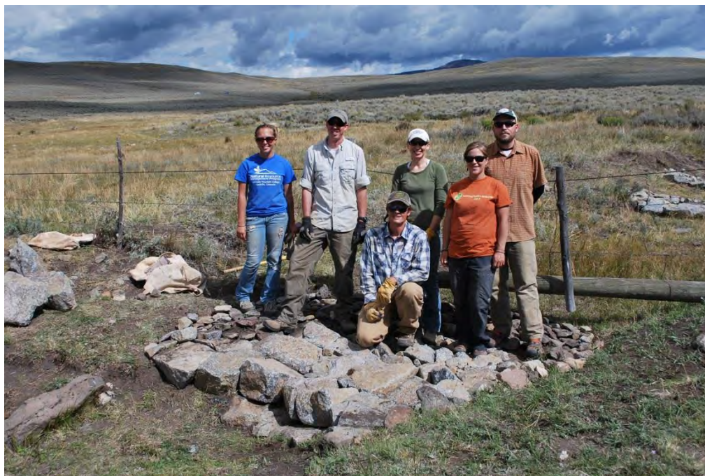
22. Wildlands Restoration Volunteer Crew Leader Clayton BonDurant (low center) and volunteers complete Zuni bowl to control a head cut on West Flat Top Mountain on US Forest Service lands, September 2014.
