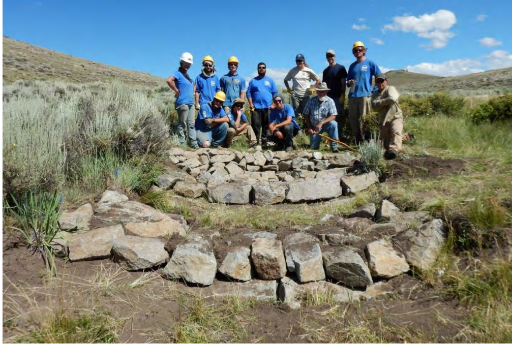
15. Western Colorado Conservation Corps, Nathan Seward, CPW, Bill Zeedyk and Shawn Conner celebrate completion of a Zuni bowl (center) with one rock dam (foreground) at Chance Gulch, August 2014. Photo: Andrew Breibart, BLM.
