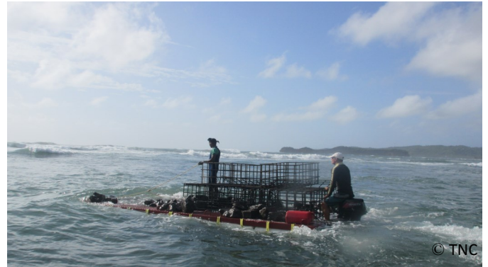
Custom made barge loaded with baskets and rocks for constructing breakwater.
