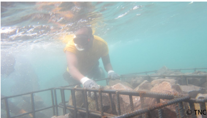
Divers carrying and packing the baskets with large armor rocks from the Telescope quarry
