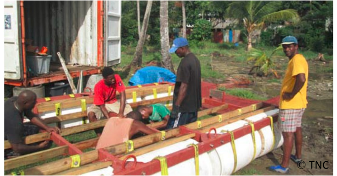
Assembly of the barge utilized to transport materials out to the reef. The barge was designed and built by Underwater Solutions with 50 gallon molasses barrels serving as pontoons
