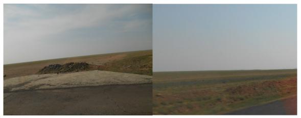
Figure 26: Berms Restricting Off-Road Traffic. Left is a single short berm blocking an existing entrance/exit point of road. Right shows a continuous berm paralleling roadway.
