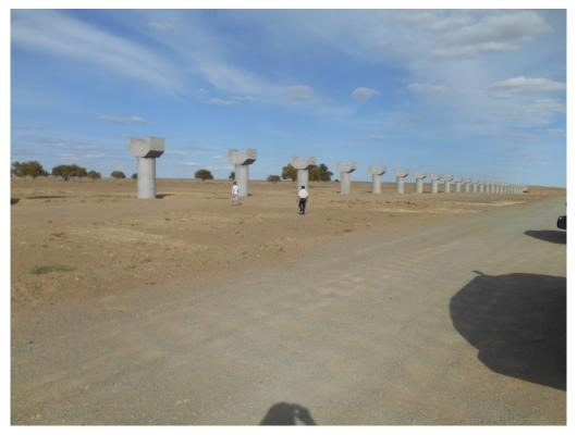
Figure 23: Wildlife Underpass on Partially Constructed Railroad
