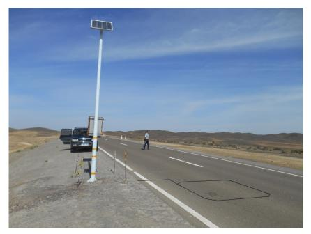
Figure 16: Induction Loop Traffic Counter on OT-GS Road (one loop darkened)
