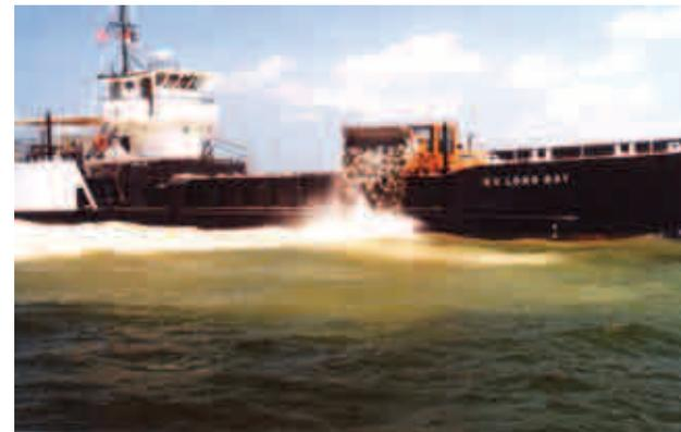
NC DMF vessel deploys riprap marl to restoration site. © NC DMF
